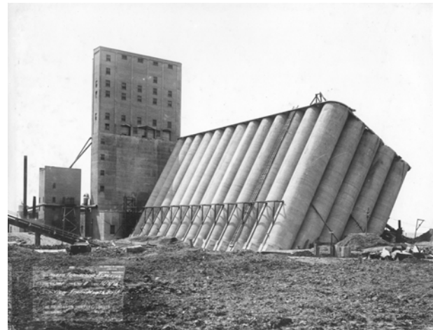
Figure 3. Binhouse after failure.
