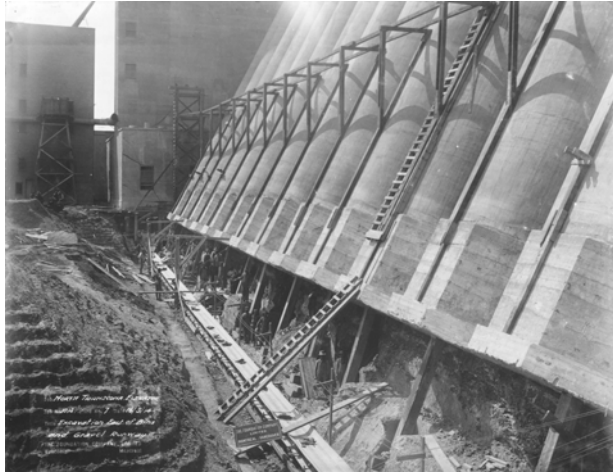
Figure 4 Excavation of the east side of the binhouse.
